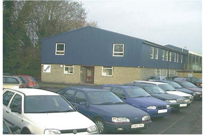
Expo Technologies main engineering and manufacturing facility
